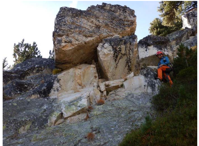
Bloc massif instable
